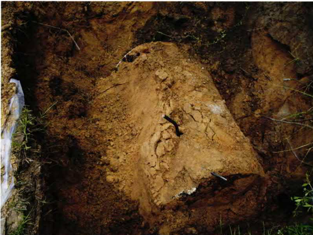
Picture 2: UST 1259Dove removal in progress.
